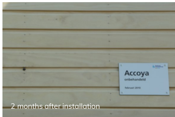
A part of the South facing façade was cladded with Accoya in April 2010, with no maintenance since. The pictures below (left to right) show this cladding in July 2010, 2012 and 2014.
