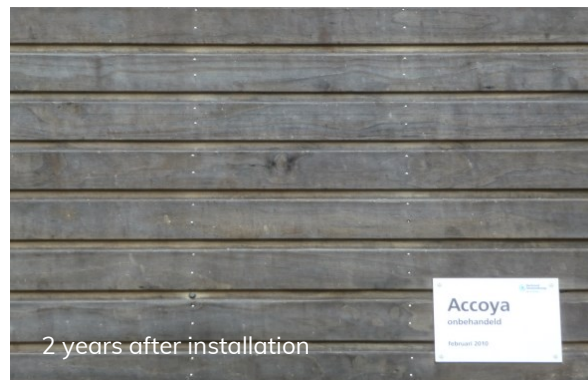
A part of the South facing façade was cladded with Accoya in April 2010, with no maintenance since. The pictures below (left to right) show this cladding in July 2010, 2012 and 2014.
