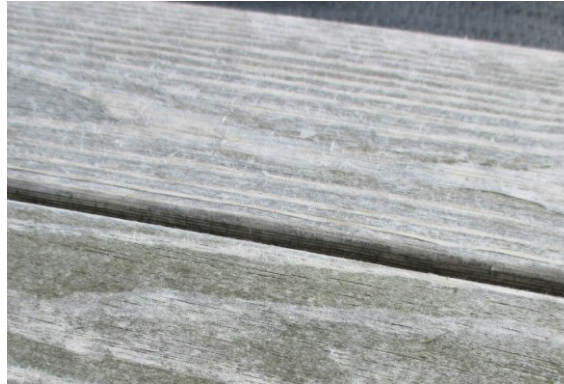
Natural occurring surface fibres on decking.
