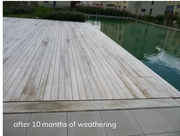
This deck in Oesingen was photographed when newly installed (left), after 10 months (middle) and after 30 months of weathering (right).
